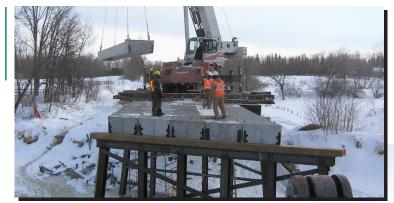
removed and replaced with a new bridge comprised of new precast concrete on new steel H piles.
